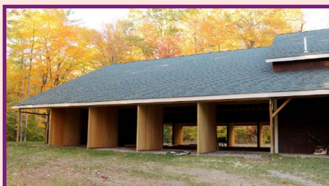
New gymnastics addition.
